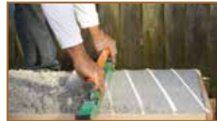
Even the surface with the screed.
