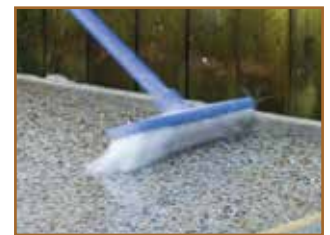
Spread the acid mix with a broom.
