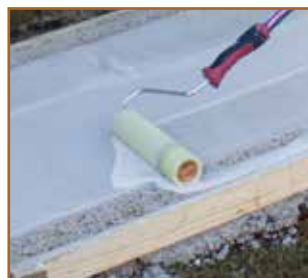
Roll over the centre of the surface in an even pattern.
