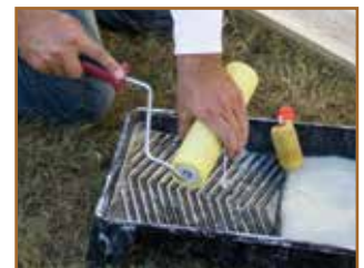
Squeeze half the water out of the roller.
