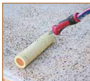
Continue rolling until the surface exposure matches the edges.
