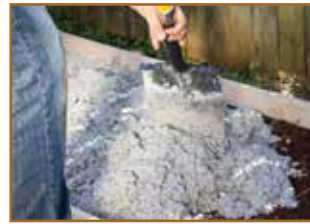
Evenly spread mix in formwork.
