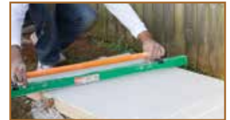
Screed until the surface is level.
