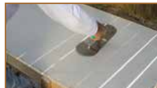
Use the float to smooth the surface
