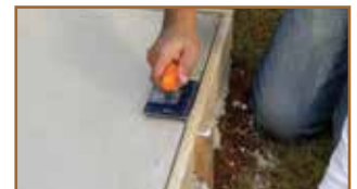
Use a jointing tool to smooth the edges.
