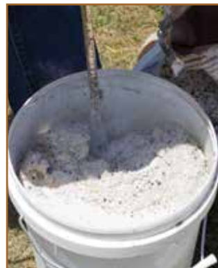
Mixing with an electric drill mixer.
