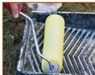
Use a paint tray to wet the large roller.
