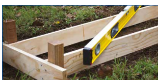
Prepare formwork
