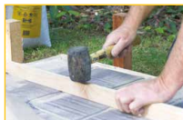
Tamp sand into paver gaps
