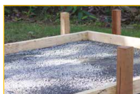
Prepare road base
