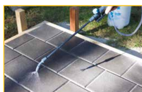
Thoroughly wet paving
