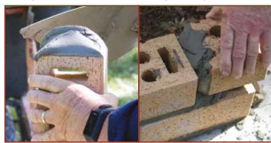
7 Put mortar on end 8 Position brick
