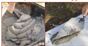
3 Mix 4 Place mortar
