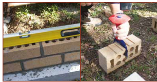
9 Check levels 10 Split for end pieces
