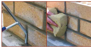
11 Rake mortar 12 Wipe down excess
