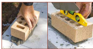
5 Lay first brick 6 Tap into place
