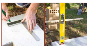
1 Mark out position 2 Check string guides
